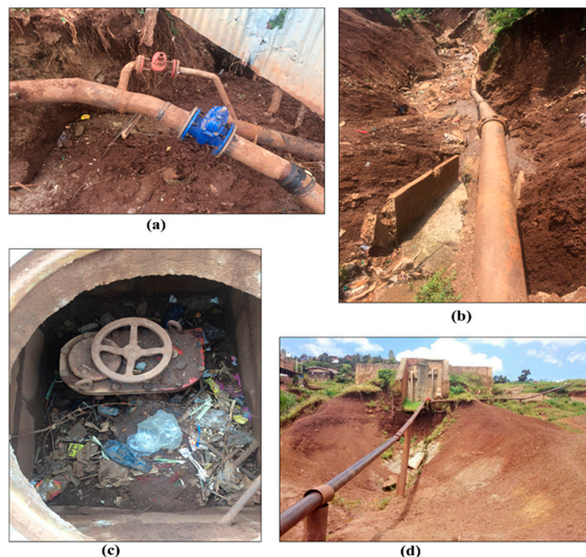
Figure 5. Vulnerability of the REGIDESO network: DN 300 pipe damaged by construction in Nfafu (a); DN 450 pipe broken by landslide in Funu (b); butterfly valve clogged with debris in Nya-kavogo (c); and secondary pipe destabilized by erosion in Kasha (d).
